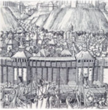
Kyiv harbour in Pochaina, the reconstruction
